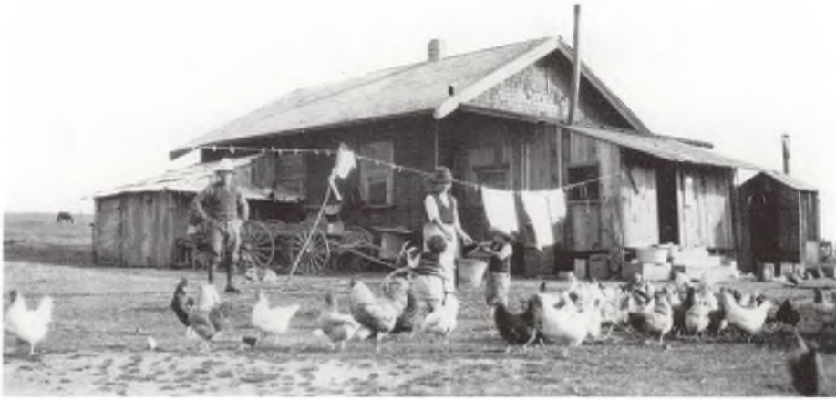
The Okidoi farmhouse complete with furo (bath), which is the tiny structure on the right-side (circa 1925).
